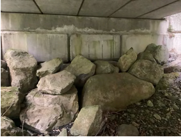
Right Bank Abutment when facing downstream
