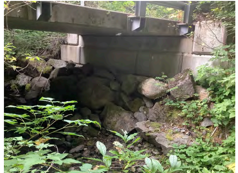
Left Bank Abutment when facing downstream
